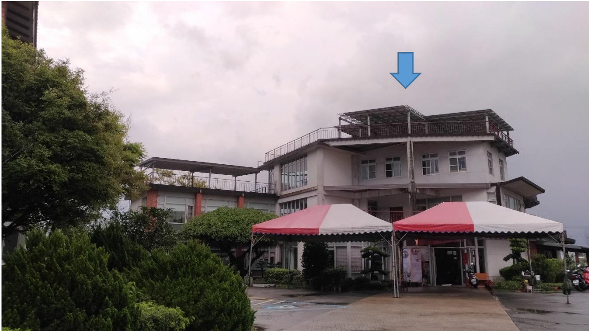
Figure 6-3. Solar panels at Julin Nursing Home
