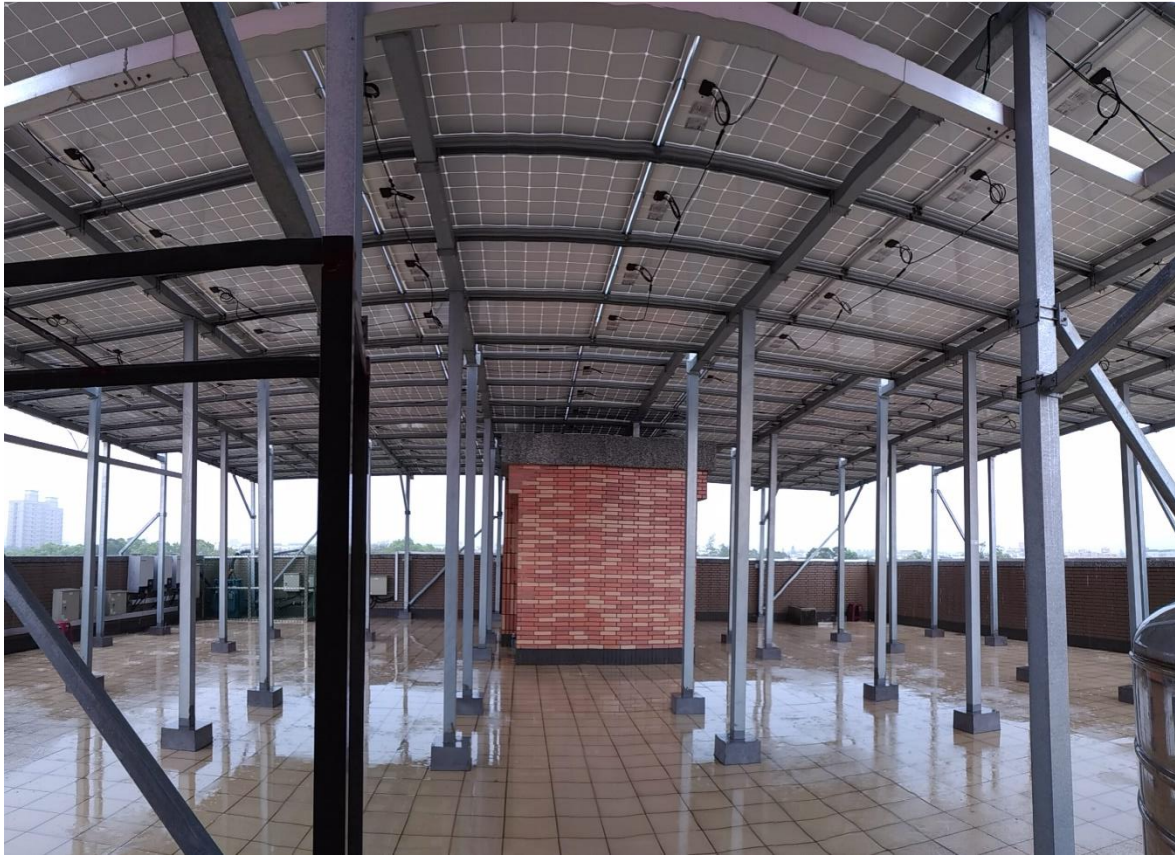
Figure 6-1. Solar panels at the Chensenmei Family Land
