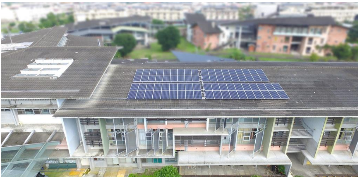
Figure 6-2. Solar panels at the St. Camillus Long-term Care Center
