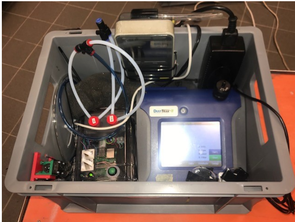
Figure 4: The set-up in the machinery room (MAR).
