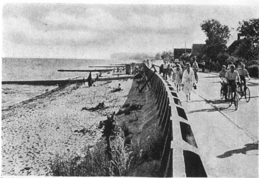
Figure 3.15: Photo from the 1960's, showing Strandvejen and the groynes placed along the beach south of the harbour (Mangor, Fuchs, & Rand, 2010).
