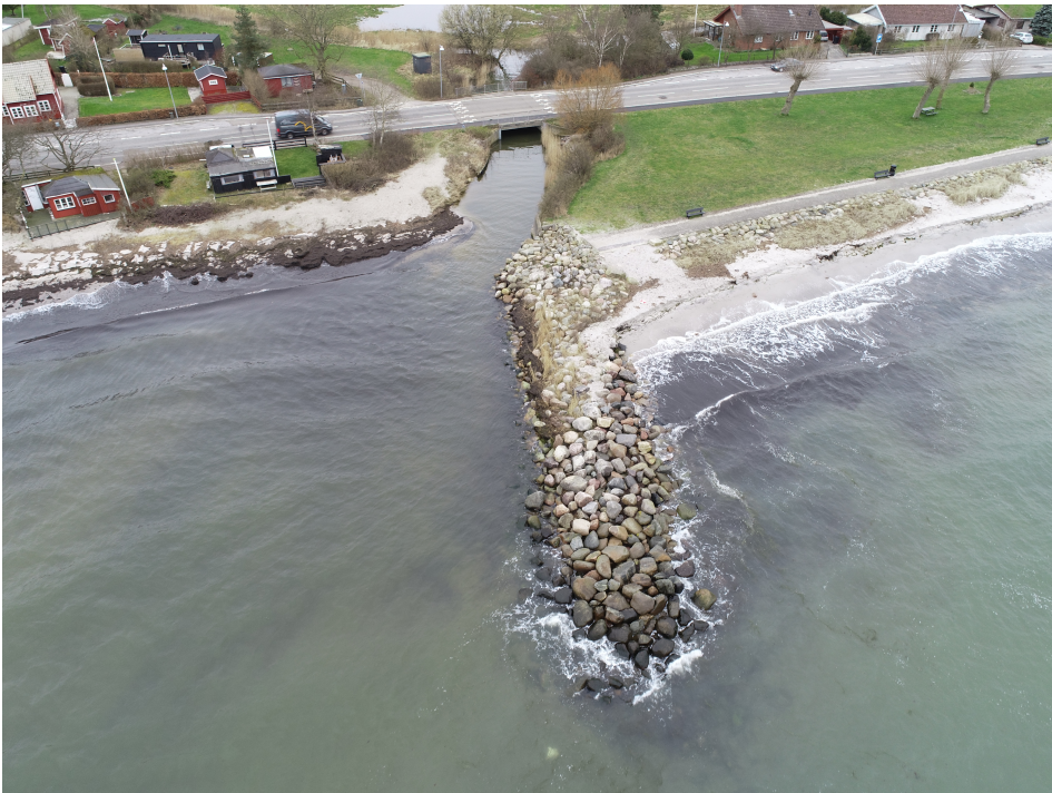
Figure 3.4: The groyne placed at the south end of the beach and just before the outlet of Faxe Creek. Photo: Danish Coastal Authority, 2020.
