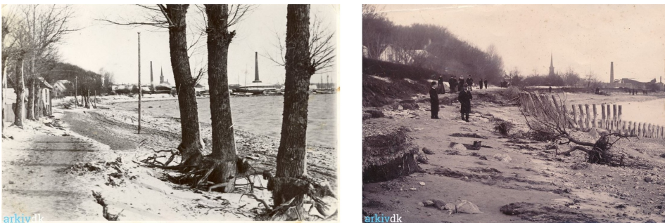
Figure 3.12: Photos showing the damages caused to the coastal area south of the harbour, during a winter storm in 1904, Left: (arkiv.dk, n.d.-b), Right: (arkiv.dk, n.d.-a).
