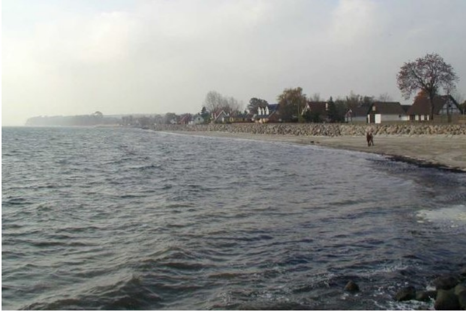
Figure 3.16: Picture from 2003, showing the recently established rock revetment along with a narrow beach strip, (COWI, 2013).
