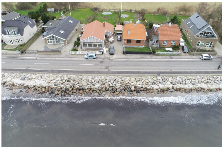
Figure 5.2: Photo from 3 March 2020 showing a section of the coast where the beach had eroded all the way to the rock revetment. Photo: Danish Coastal Authority, 2020.
