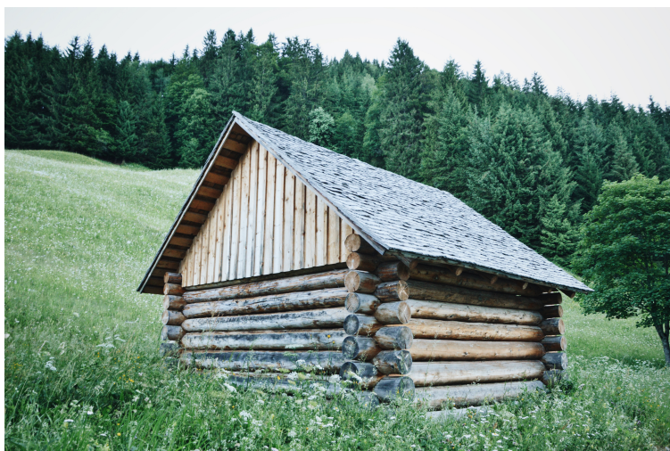
Figure 1: Rooftop by Linda Erwe
