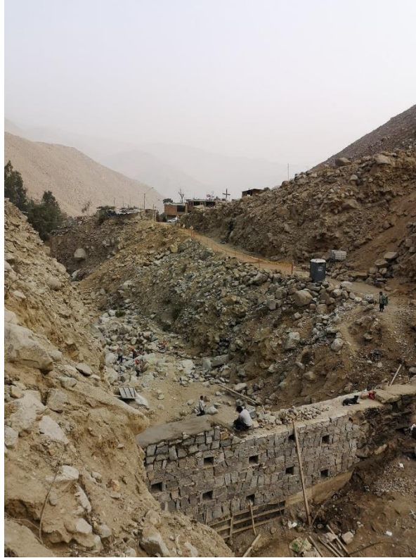
Figure 13: Construction of a rock wall in a quebrada in the arid transition zone. Photo: Author's own.
