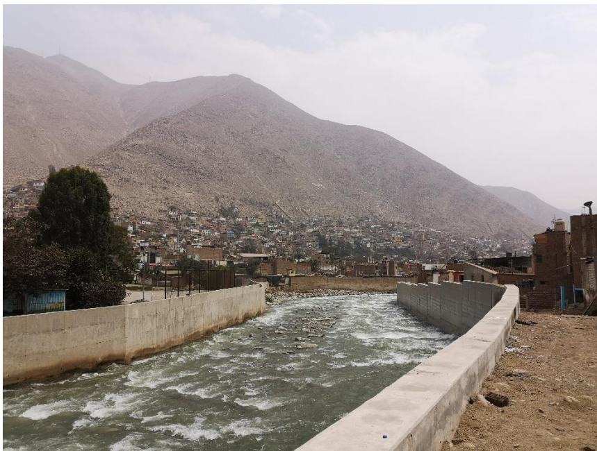
Figure 12: Channelisation of the Rimac river in the arid transition zone. Photo: Author's own.
