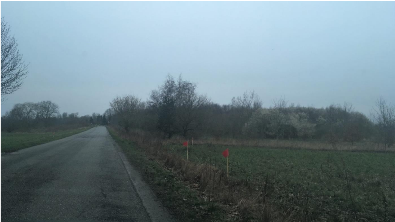
Figure 4: Red flags outline the future path of the pipeline near Stig's residence. Photo by the author.
