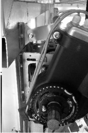
(a) Figure shows installation of the operator before mounting the sensor.
