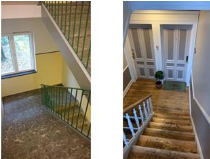
Figure 1: Functional staircases from two different locations. Photographed in September 2019
