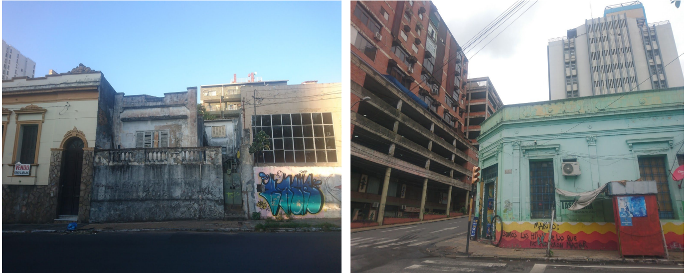
Figure 15-16: Abandoned and ill-maintained buildings in HCA. Source: the author
