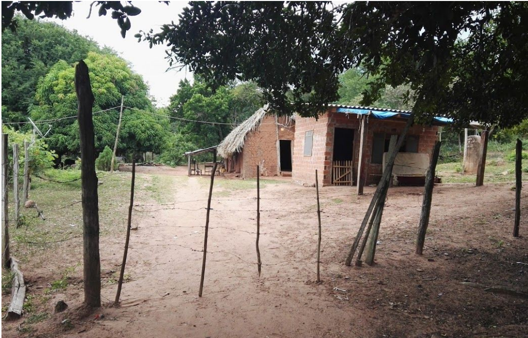
Figure 11: An additional room built in brick | Private picture, 2020
