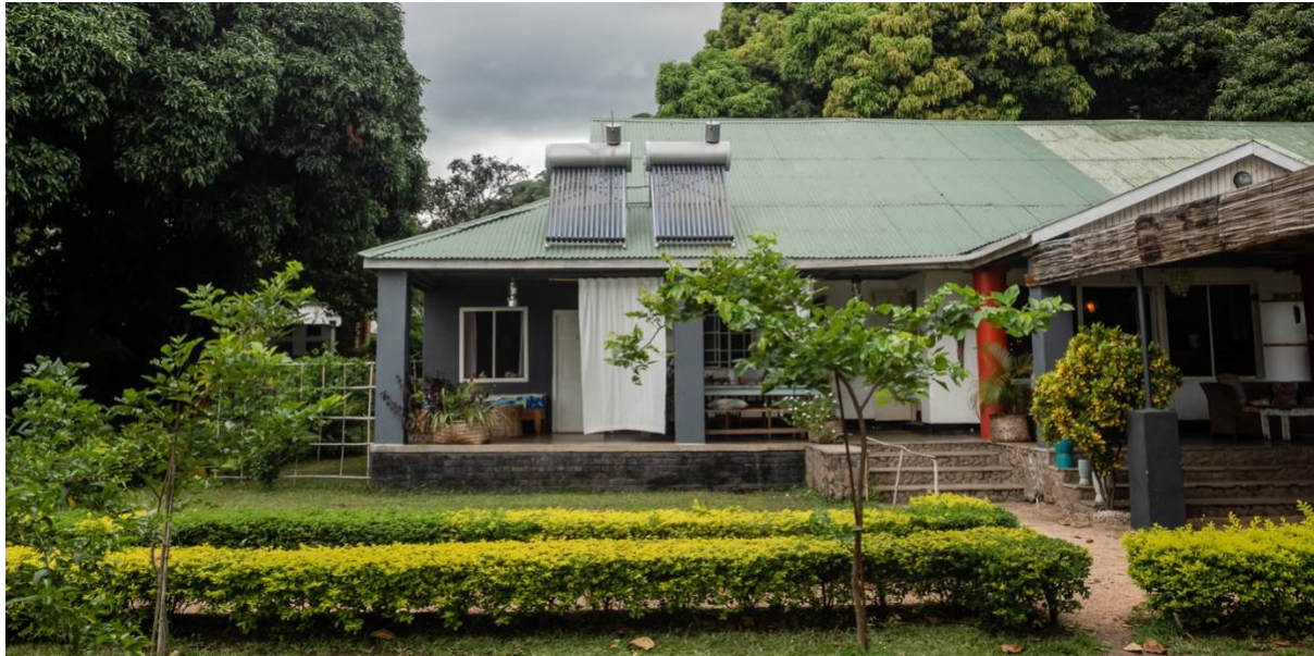
Picture 6: Solar energy at the roof of Monkey Bay beach lodge. Monkey Bay. Zoe Elsner.
