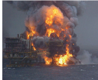
Figure 6 - Pipe Alpha, after the explosion (Whitmeyer & Wilcutt, 2013)
