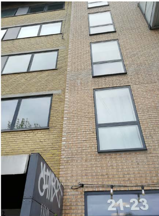
Figure 64: Reference for the combination of old and new fabric. The particular surface pattern of new bricks creates an interesting texture and a nice contrast to the existing brick wall. New windows adopt the frame colour and width of the existing windows, while the new windows extend to the floor.
