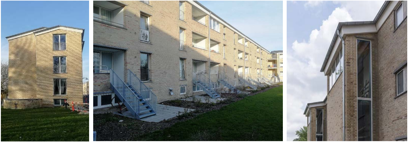
Figure 45: Tingbjerg: Small gable wall with French balconies (left), new staircase access and private gardens for apartments at ground floor (middle), Integrated elevators with slight extension of staircase walls (right)
