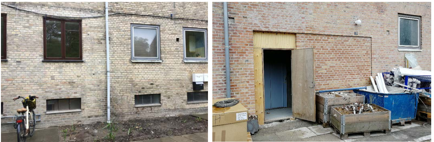
Figure 35: Lundevænget: New and old windows (1980s) next to each other (left), Entrance with recessed brick wall to mark entrance with elevators (right)
