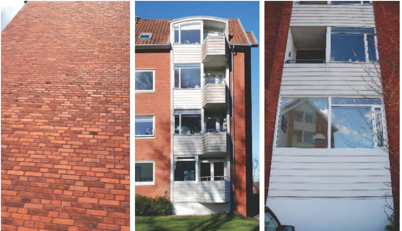
Figure 26: Højstrupparken: Insulated gable wall with a mix of old and new stones (left), Mock-up of new balcony and oriel on ground floor (middle); Illustration of covered gable balcony on ground floor (right)
