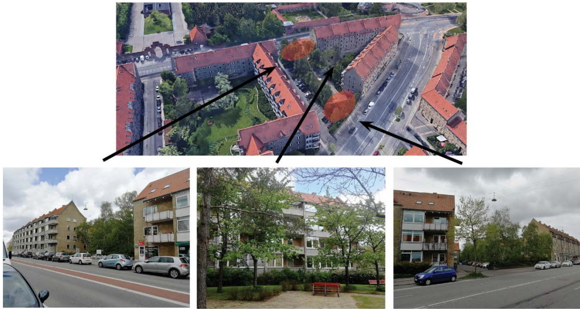
Figure 53: Pictures from the project site
