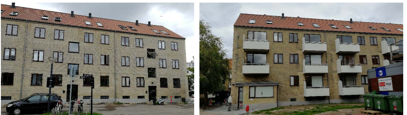
Figure 36: Lundevænget: Renovated facades with new windows and new roof + roof apartments
