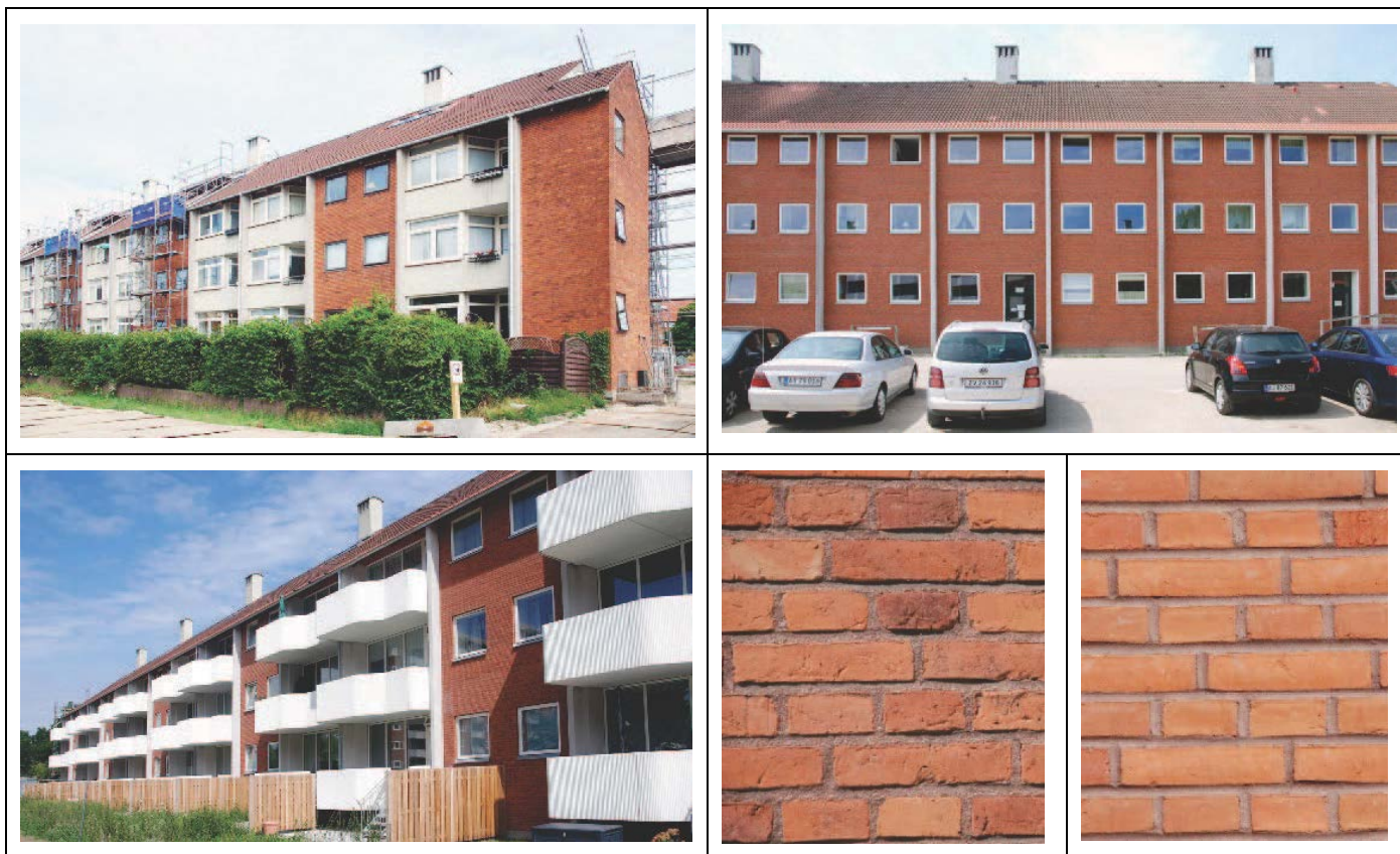
Figure 29: Brøndbyparken Afd1: Original balconies (top left) and new balconies (down left), Extended roof with new tiles (top right), Original tiles (bottom middle) and new tiles (bottom right) of the insulated outer wall
