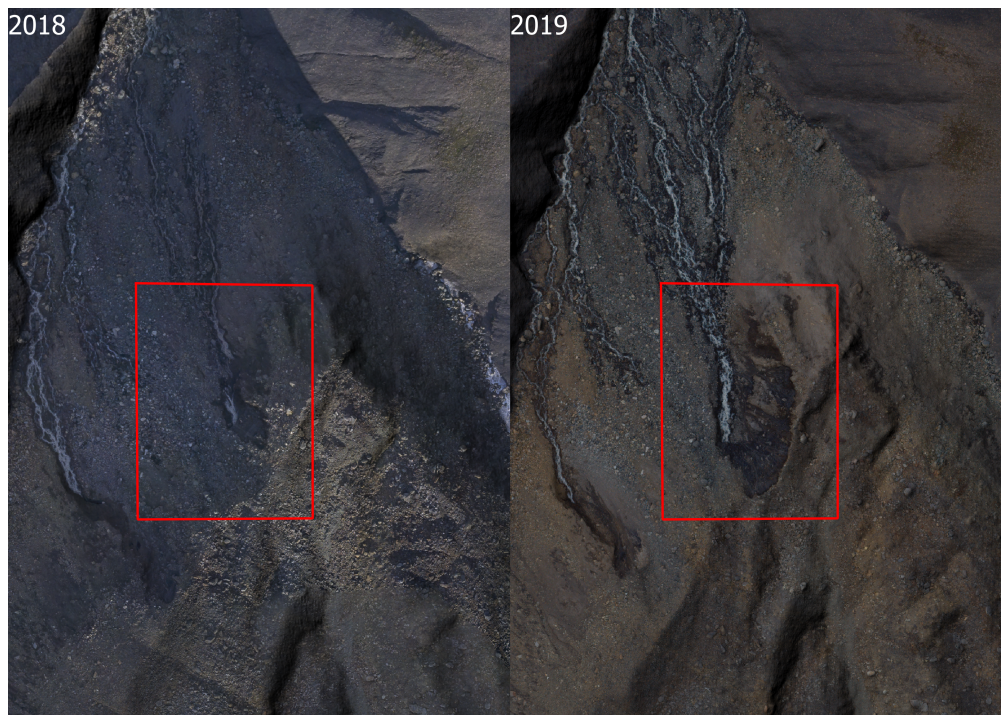
Figure 8: Collapse of a meltwater tunnel
