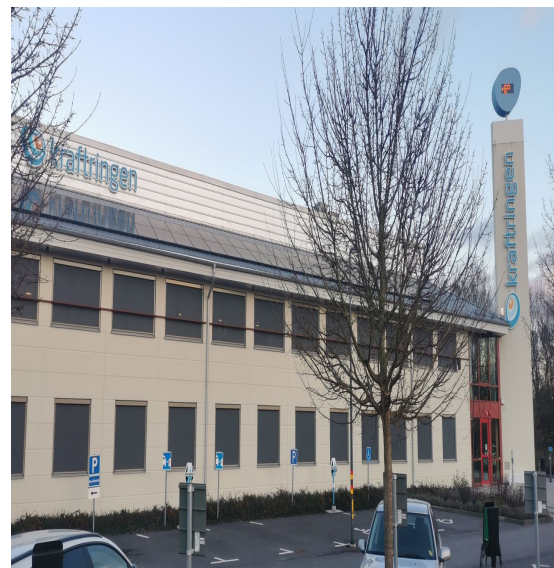
Figure 1: Solar panels installed on the rooftop of Kraftringen where the work was carried on.
