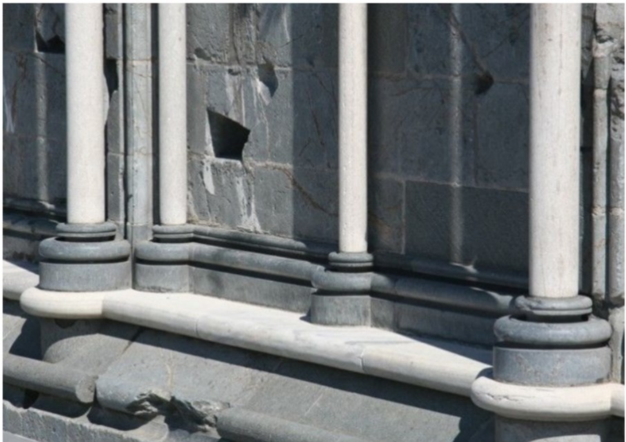
Figure 3. Columns made of marble from Allmenningen, in the Nidaros Cathedral in Trondheim. Photo from Tom Heldal, NGU.
