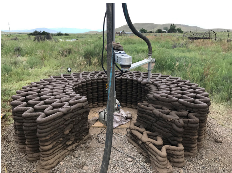
Fig. 3 Portable SCARA robot designed for in-situ printing. ©2019 Emerging Objects
