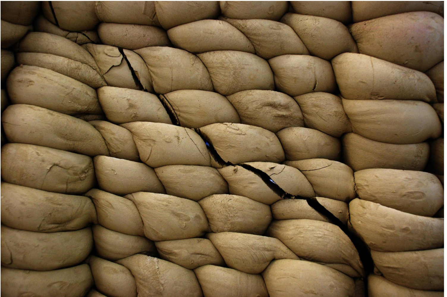
Fig. 21 Cracks developed during drying due to uneven shrinkage.
