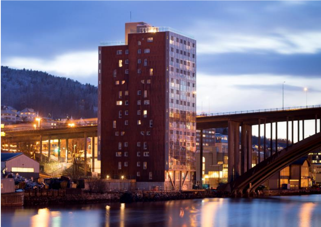
Figure 1. The 49 m high Treet (The Tree) apartment block in Bergen, Norway, was completed in 2015 and is one of the tallest cross-laminated timber structures in the world (WSP, 2017). Photo: David Valldeby, published with permission from the copyright holder.
