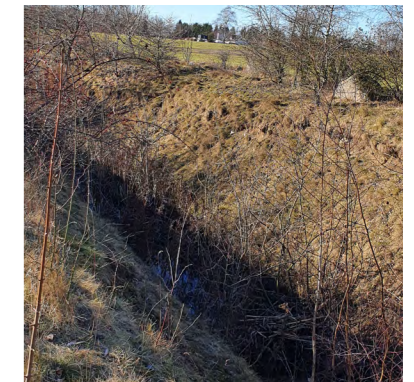
6 Ditches for storm water management
