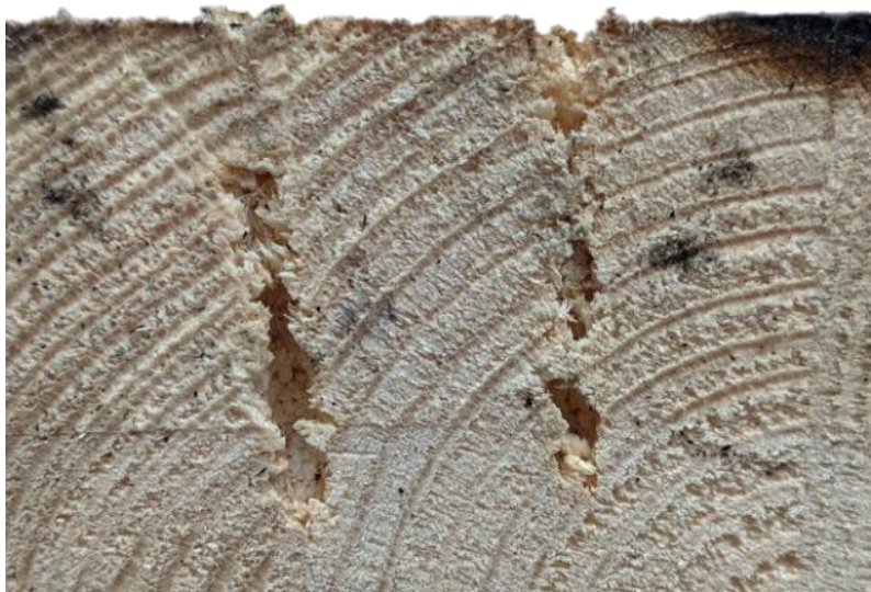
Figure 37. Bores in the 4th test showing discoloration
