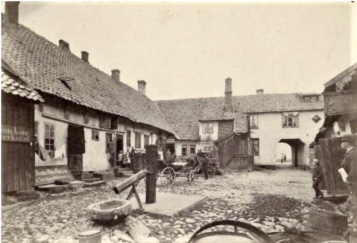
Figure 38: the yard of Trappska gården in the 1890s. Photographer Alfred B. Nilson. Helsingborgs museum.
