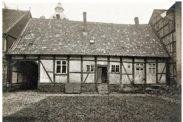
Figure 29: Kullagatan 3 in 1921 from the yard. Helsingborgs museum.
