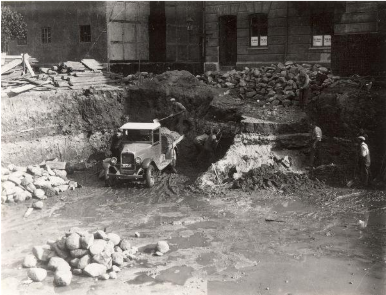
Figure 56: excavation of the foundations for the HD House, 1929. Helsingborgs museum.
