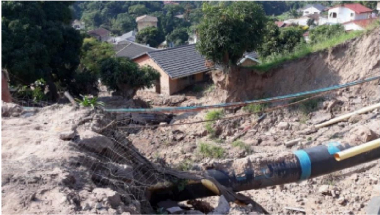
Figure 6.6. Impact Flooding in Westville: eThekweni Municipality Annual Report 2018/ 2019
