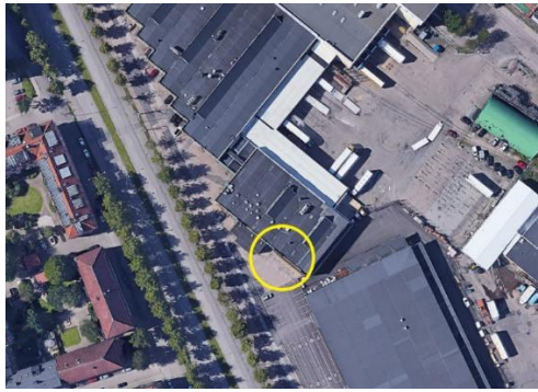
Figure 7: Aerial view of the office yellow circle.
