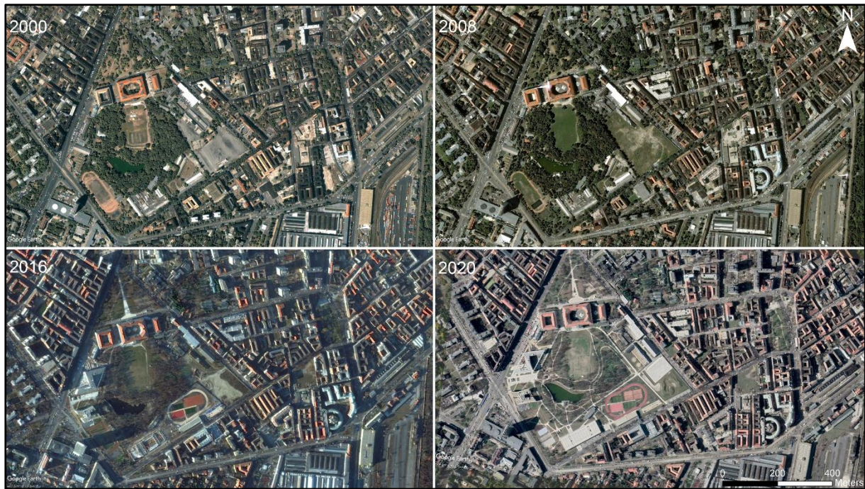
Figure 4. Historical change of the National University of Public Service campus redevelopment area. Source: Google Earth, n.d. b; own editing
