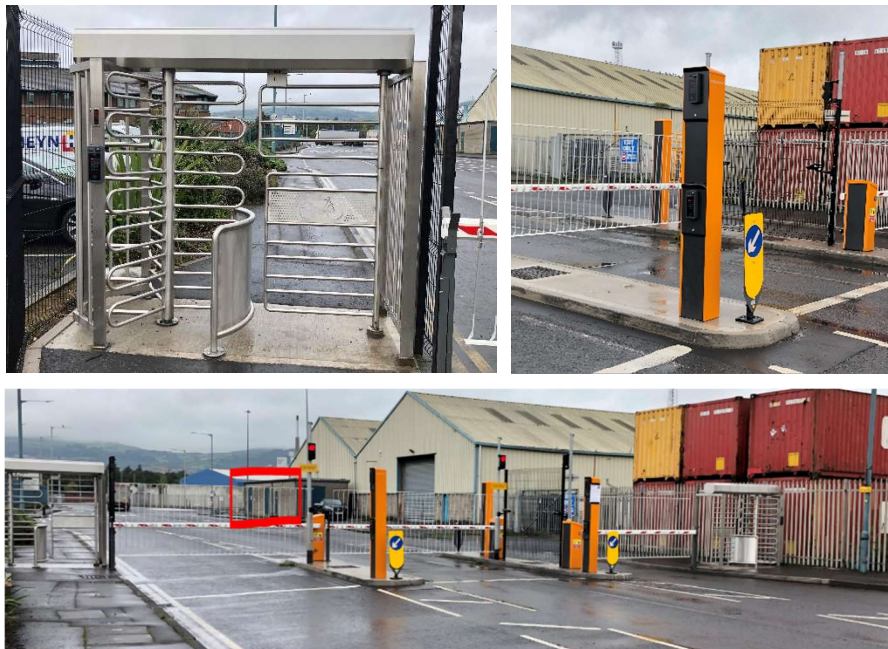
Figure 2.9 a-c, Intercom devices mounted in the windy conditions of a European harbor.
