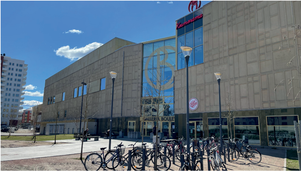
Entrance facing the cultural district with poor transparency of the facade, sending a message to people that they can not go through
