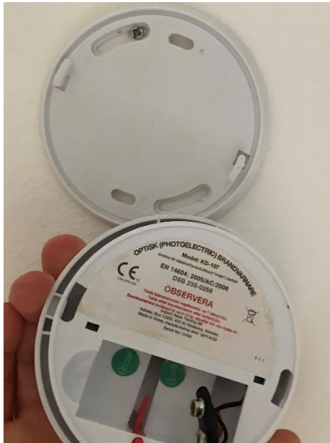
Figure 36 A fire alarm which is fitted using a bayonet mount onto a base plate. (Michael Lindberg)
