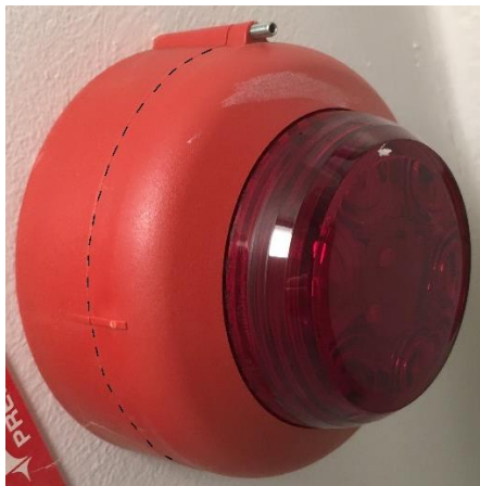
Figure 42 A fire alarm fitted with a bayonet mount and a securing screw. The cover is two-parted and black stripes was added afterwards to display the parting-line. (Otto Reerslev)
