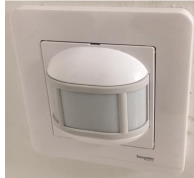
Figure 41 A permanently wall mounted motion detector capable of detecting movement in front of it. The outer cover may be detached by prying it off using a screwdriver. (Otto Reerslev)
