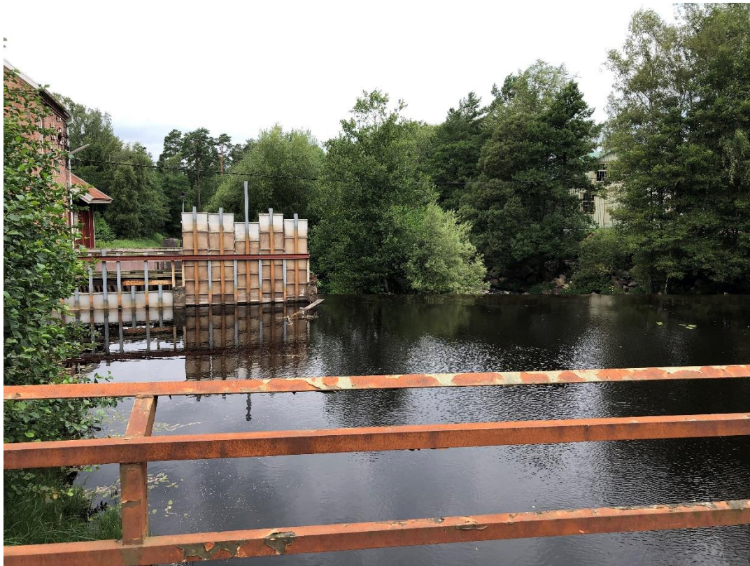
Figure C. 4 Storån (downstream) near river station 70184, Bridge code: B6
