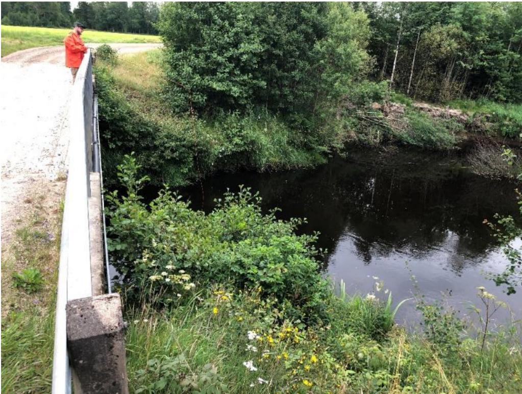
Figure C. 2 Storån near river station 56260, Bridge code: B5
