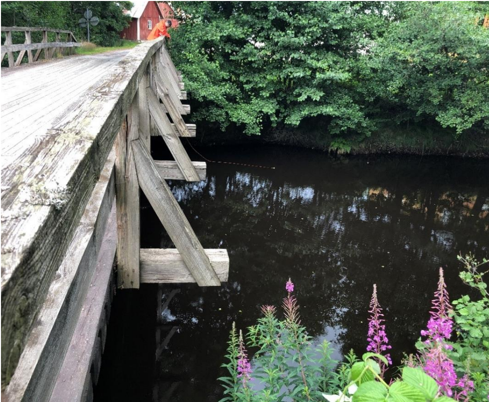
Figure C. 1 Storån near river station 46536, Bridge code: B4
