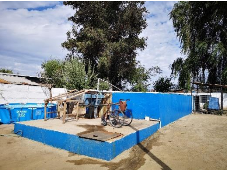
Figure 33. The existing treatment plant today that consists of one reactor piscine (Source: Author).
