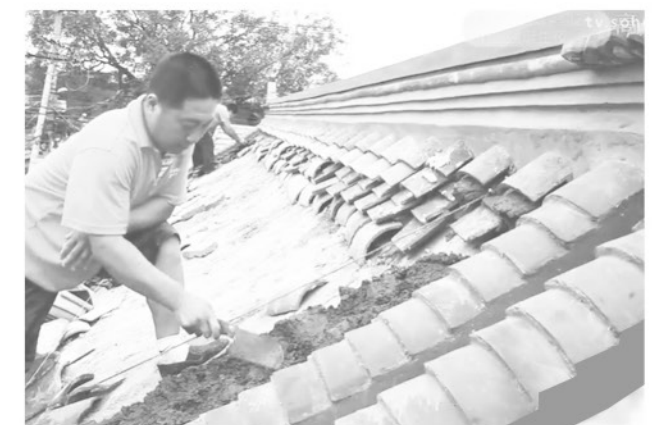
cover 15cm thickness tibia and place the tiles
