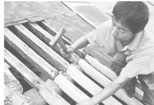
nail wooden rafters
