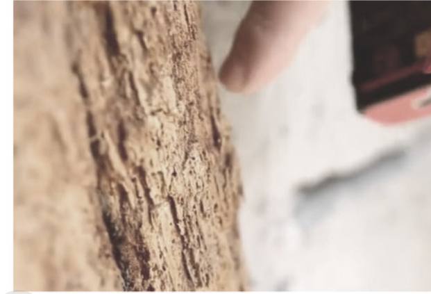
D PROBLEMS in restoring beam & column Decayed
