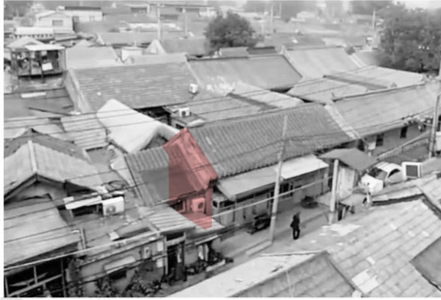
B THE PROBLEM in restoring shared wall Bad sound insulation
