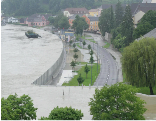
Seawall in Grein, Austria Images source: www.reddit.com/r/pics/comments/1sl1fb/mobile_flood_wall_in_austria_amazing_feat_of/
