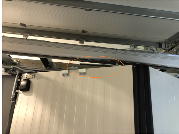
Figure 3.9: Arm connecting door to driving chain in horizontal position (4 seconds into the opening cycle).
