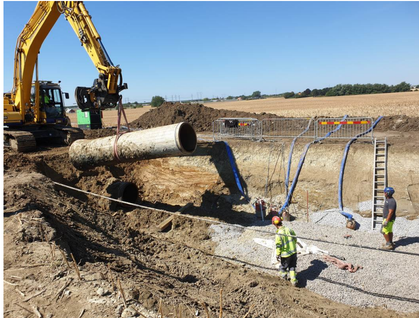
Figure 4: Repair of the pipe break of the major supply pipe from Vombverket. Photo by Sydvatten AB.
