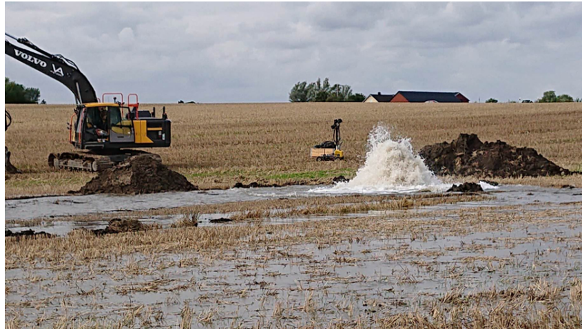
Figure 2: The pipe break that occurred between Teckomatorp and Västra Strö. Photo by Sydsvatten AB.
