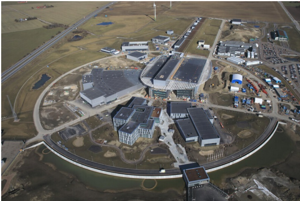
Figure 1.1: Aerial view of the ESS construction site [5].
