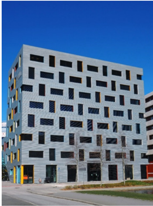
facade B in Jättåvågen. Two primary visual elements seen on the right side. Photo: S. M. Sivertsen
