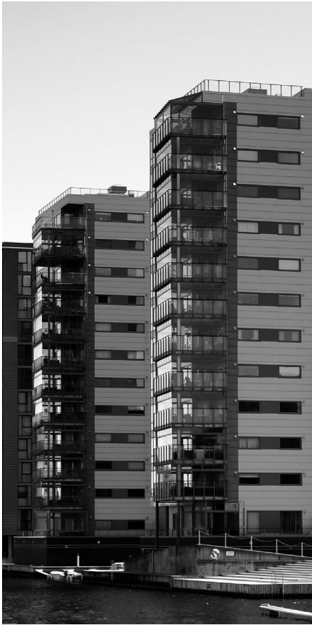
Contemporary architecture in Stavanger, Norway. (Photo: S. M. Sivertsen)
