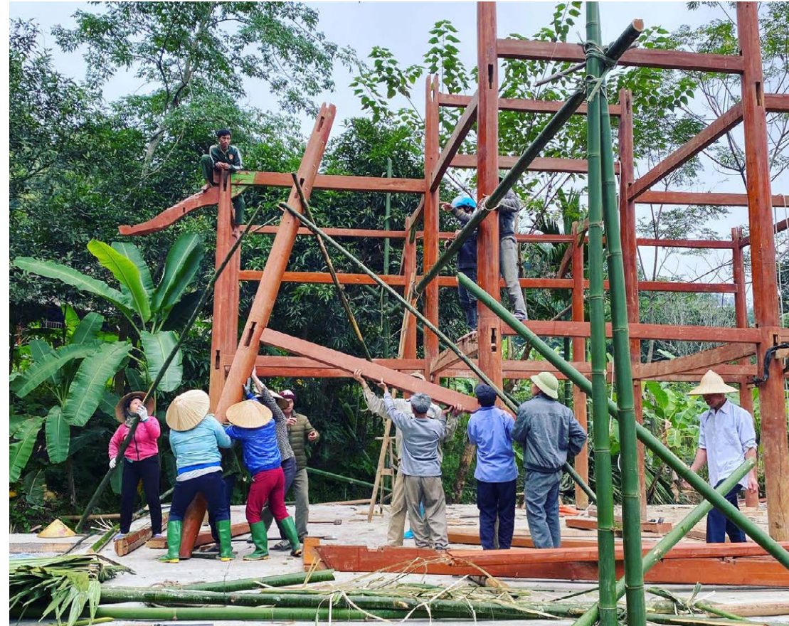
Local people re-erecting the house from old frame ( image: Jack Ecolodge)
