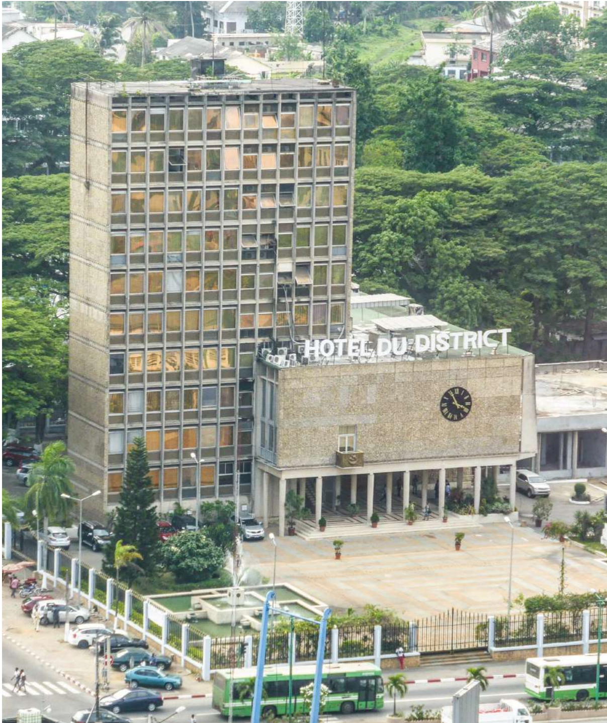
2.18 Hôtel du District in Abidjan, Côte d'Ivoire. Built between 1954-1956 by BEHC Henri Choumette with A. Laget.
