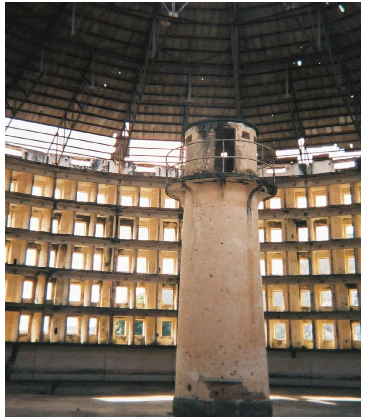
5.3 View from inside Presidio Modelo, in Cuba, a model prison with panopticon design, in which the guard is situated in the central tower, with all cells visible, located around it.
