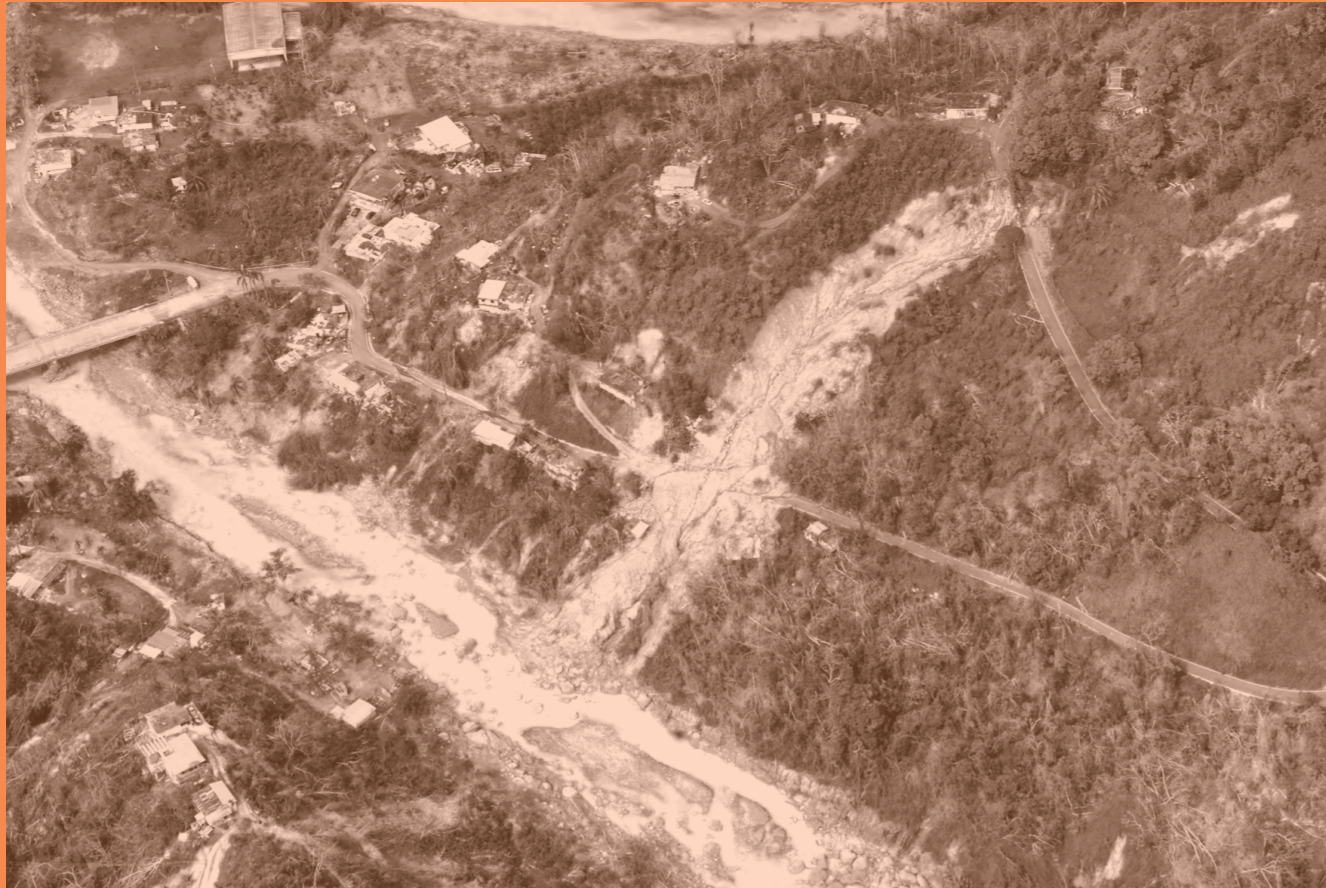
66 Landslides in Puerto Rico
