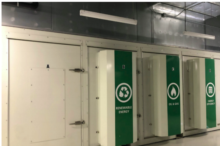
Figure 1.11: Natural-gas-burning microturbine system with heat exchanger form the backbone of the microgrid for the office building and data center [10].
