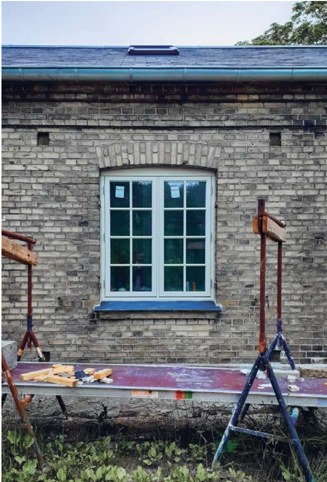
Figure 148 Continuous work is conducted renovating historical buildings on site
