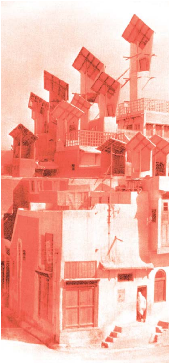
Figure 01 The air-conditioners of Hyderabad Sind which was part of The Architecture Without Architects project
