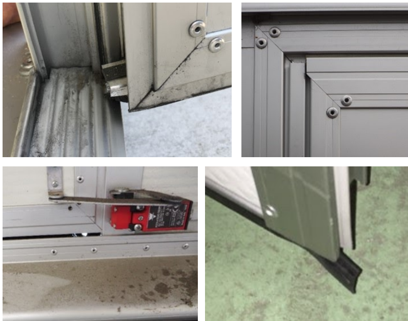
Figure 4.15 - Corner problems with the roton profile used in Passdoors.
