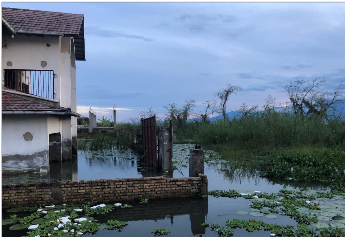
Figure 4: House flooded by Lake Tanganyika (Own photo)
