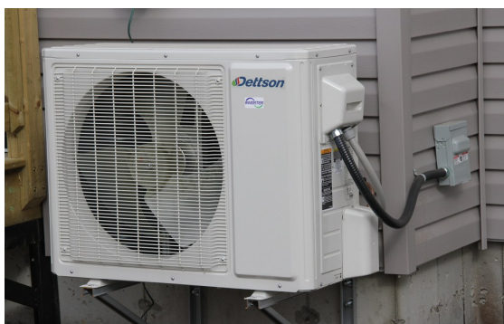
An air source heat pump outside private housing (Unknown Author, licensed under CC BY-SA-NC)
