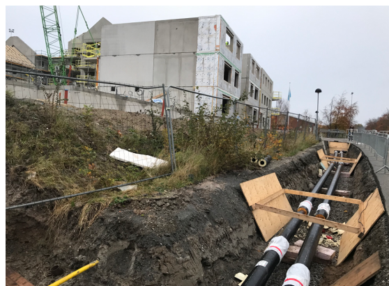
District heating pipes for a new building in Lund (Own Picture)
