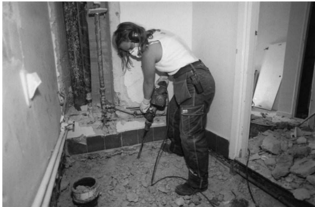
A participant renovating the bathroom (Edström).
