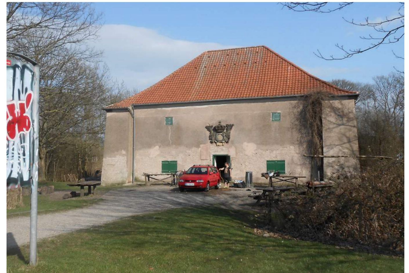
Photos of the old powder houses on the Vold, taken on my second visit in spring 2018. These are a sample of the local structures that have been turned into dwellings over the years.
