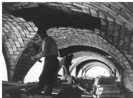
Figure 9. The making of the brick vaults.
