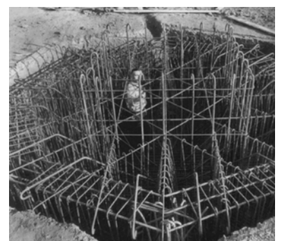
Figure 10. The construction of a plinth.
