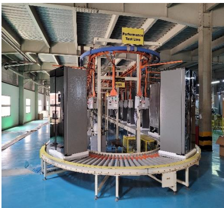
Figure 9: Performance Testing Line
