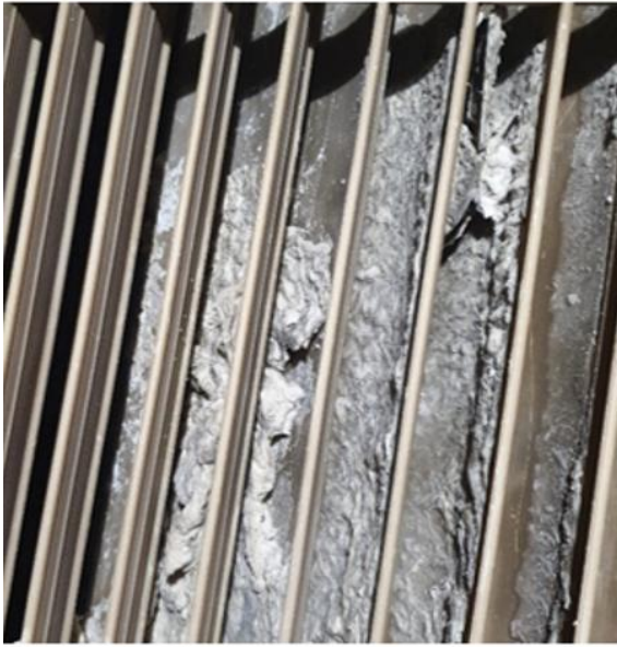
(a) Scaling in droplet separator
