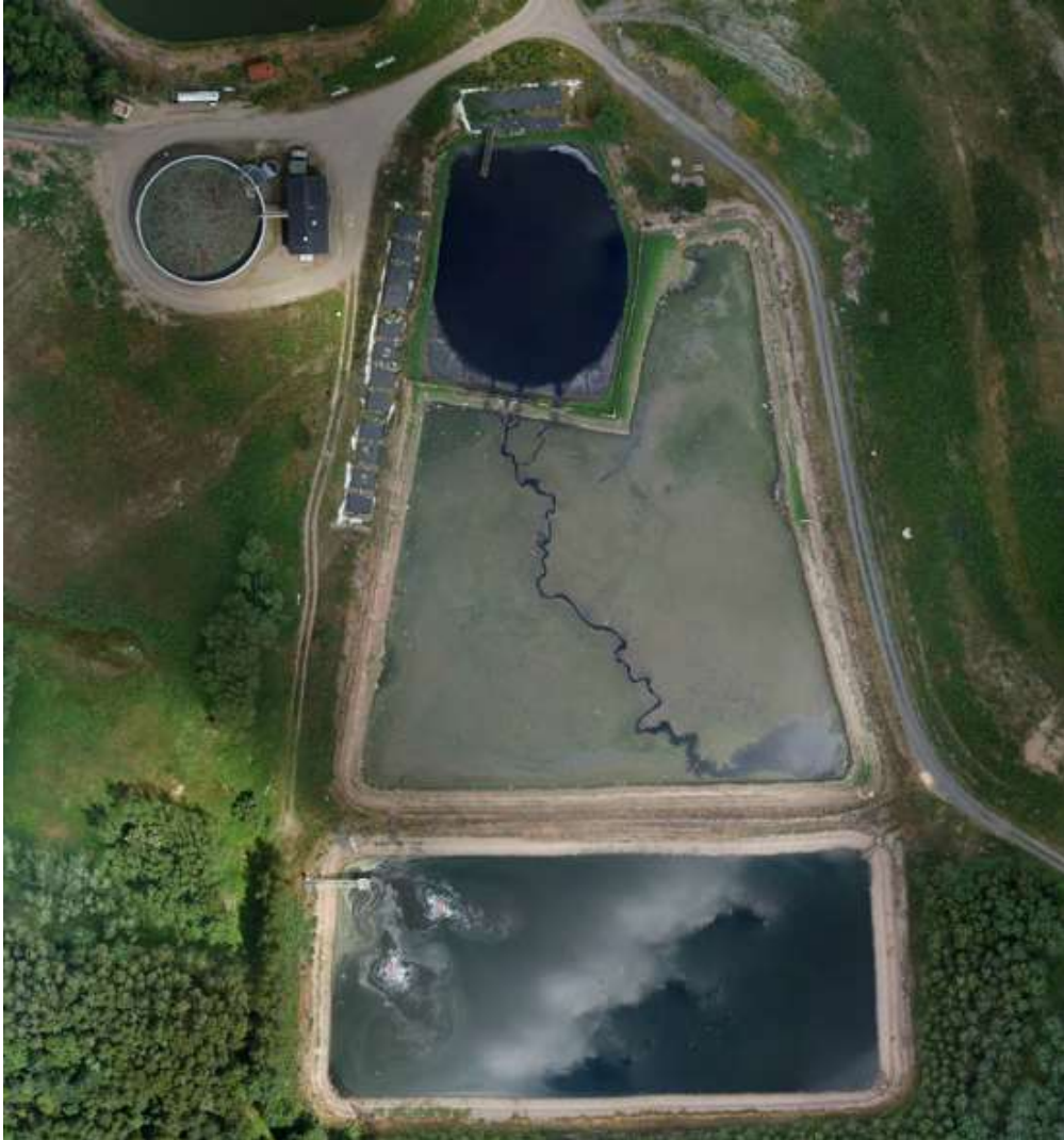
Figure 2.2. Leachate storage ponds and the treatment plant (top left)
