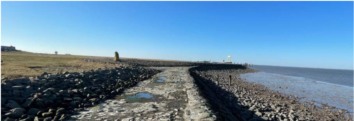
Figure 7. Revetment on Hallig Hooge. Stone revetment on the northern side of Hooge with the ferry dock in the background. The revetment is around 2 meters wide and paves the Hallig edge. Picture taken on the 27 th of February 2022. Own work.
