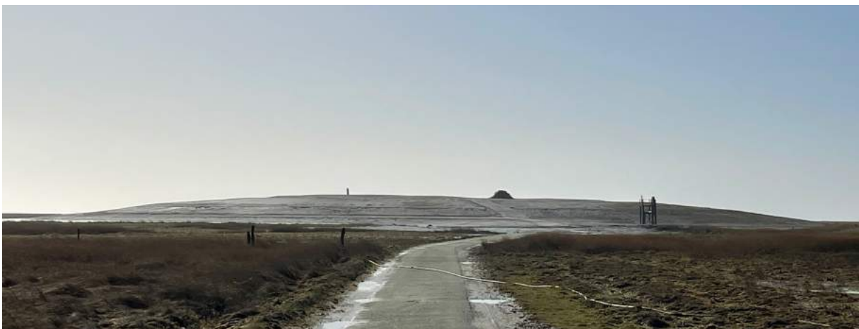
Figure 10. Reinforced Treuberg terp. The picture shows the reinforced Treuberg terp on Langeneß which is now 5,9m high. Picture taken on the 23 rd of February 2022. Own work.
