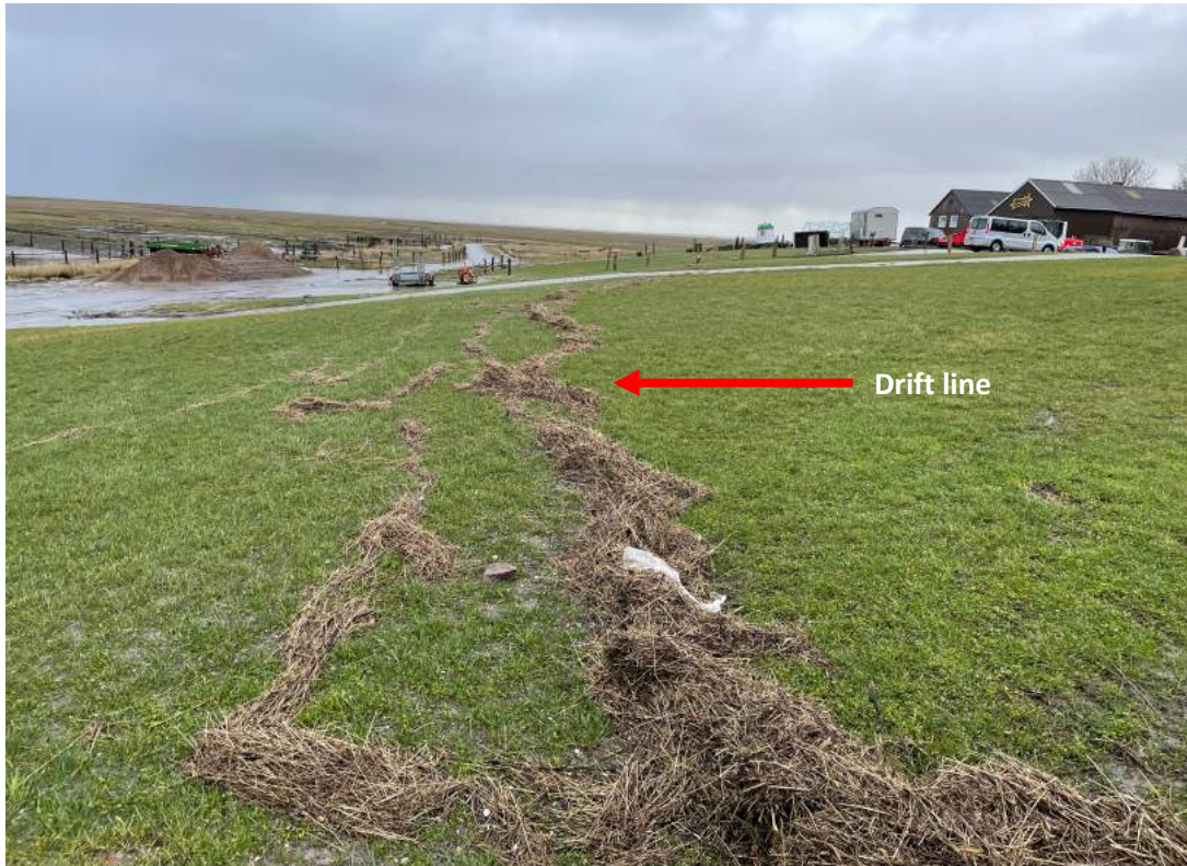
Figure 12. Drift line on the northern side of Hanswarft. Drift line on the reinforced northern side of Hanswarft on Hooge. The drift line is half way up the terp. Picture taken on the 25 th of February 2022. Own work.
