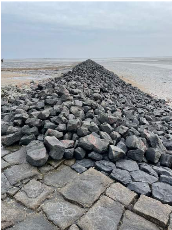
Figure 8. Groyne on Langeneß. This picture shows a groyne made of stone on Langeneß. It is around 30 meters long and 4 meters wide. It vertically protrudes from a Hallig . By protruding into the ocean, groynes interrupt the water flow thus reducing erosion and water speed. Picture taken on the 22 nd of February 2022. Own work.
