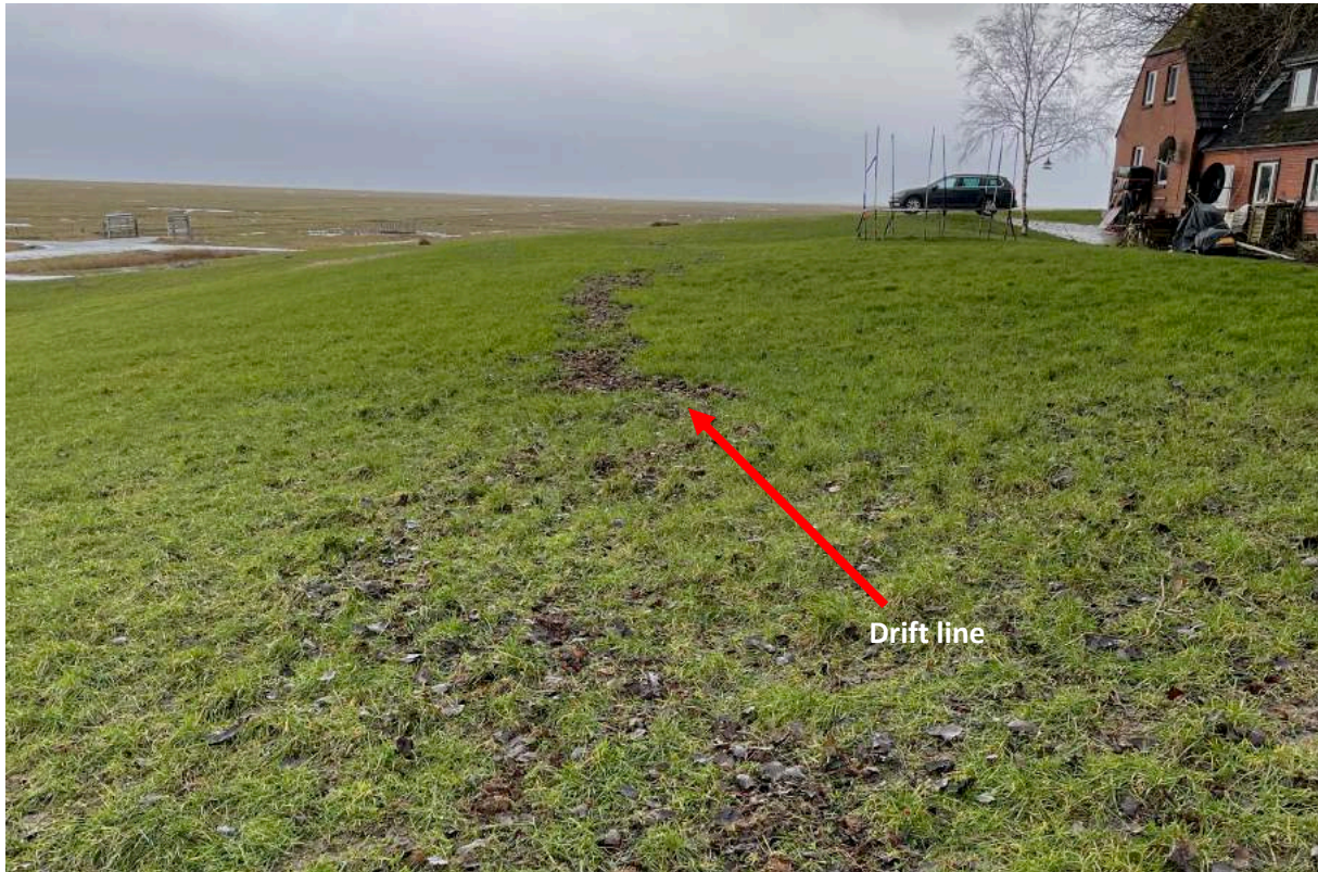
Figure 13. Drift line on the eastern side of Hanswarft. The picture shows the drift line on the not reinforced, eastern side of Hanswarft on Hooge. The drift line is three-quarter up the terp. Picture taken on the 25 th of February 2022. Own work.
