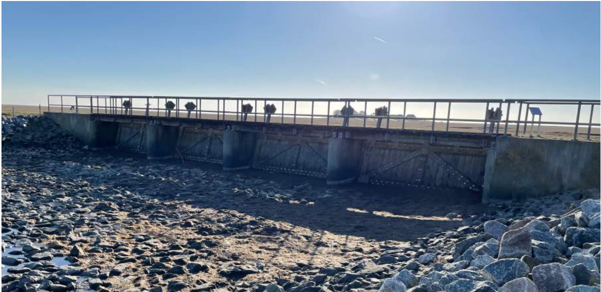
Figure 9. Sluice on Hallig Hooge. This picture shows a closed sluice on Hallig Hooge. This sluice controls the water levels of the biggest tidal creek on Hooge. Picture taken on the 27 th of February 2022. Own work.
