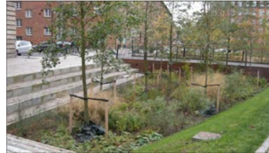
“Danish rainforest” Tåsinge Plads in Copenhagen has been rebuilt to be able to store larger amounts of rainfall as part of Copenhagen’s cloudburst plan. (17)
